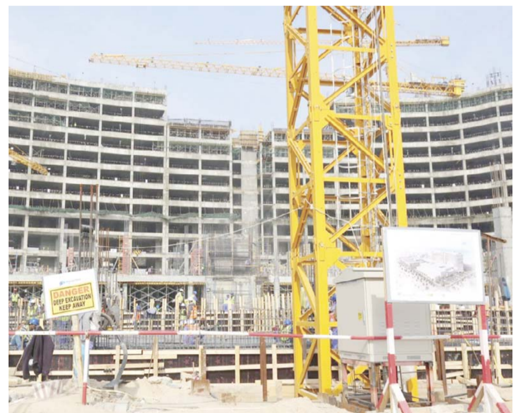
KUWAIT: Ongoing construction works at the new Sabah Hospital's project. — KUNA
