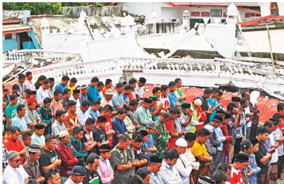
TRINGGADING, ACEH PROVINCE, Indonesia: Survivors perform Friday prayer at a Jami Quba mosque which was severely damaged during Wednesday's earthquake on Friday, Dec 9, 2016. — AP
