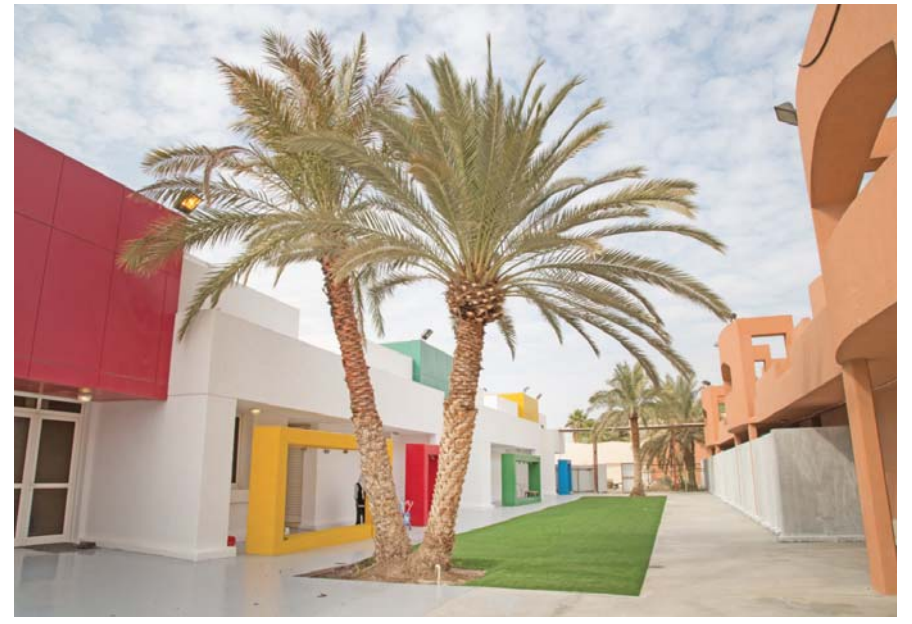
The renovated houses.
