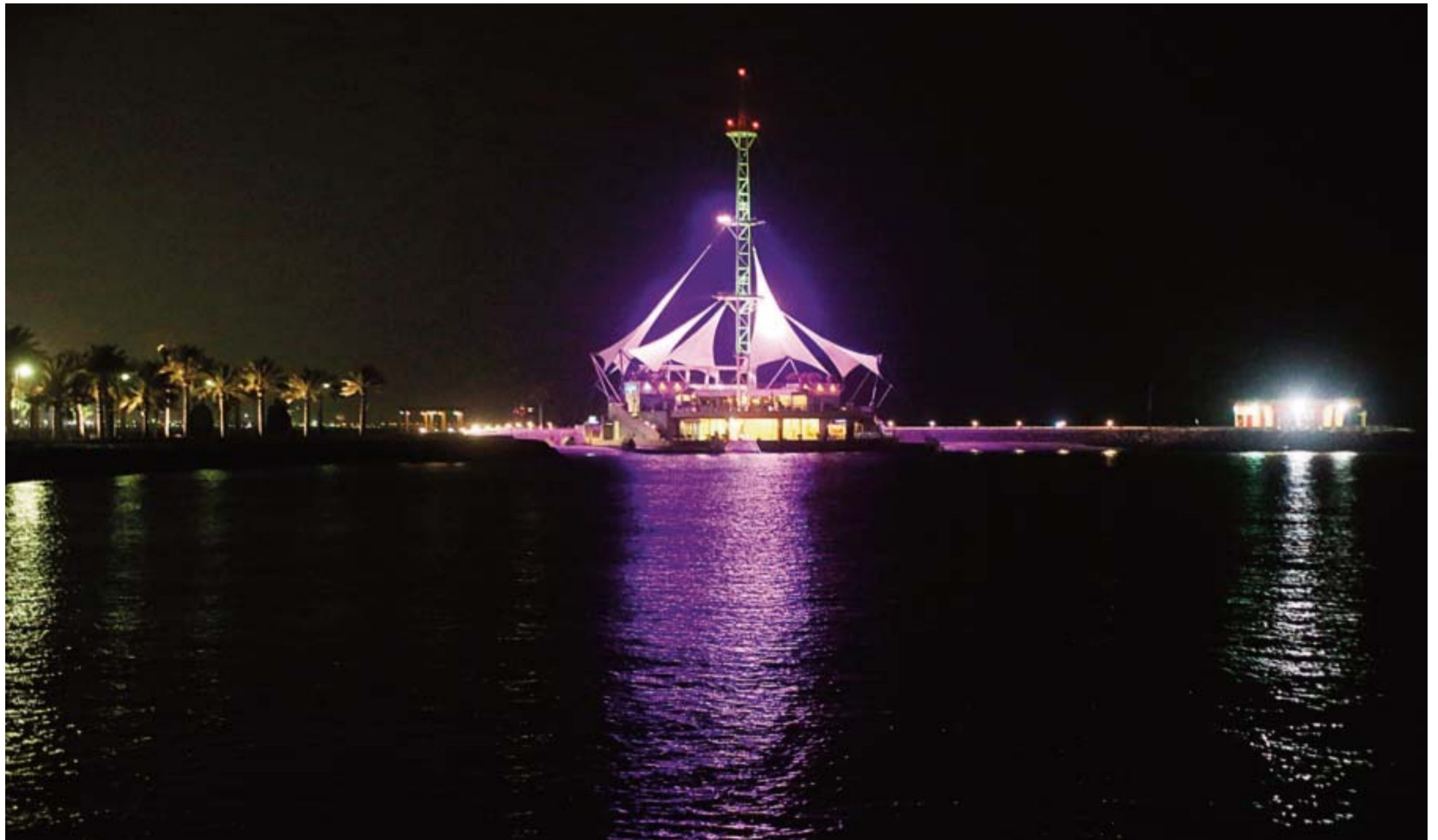
KUWAIT: The 'Marina Waves'; a landmark structure located in the Marina Crescent in Salmiya. —Photo by Yasser Al-Zayyat
