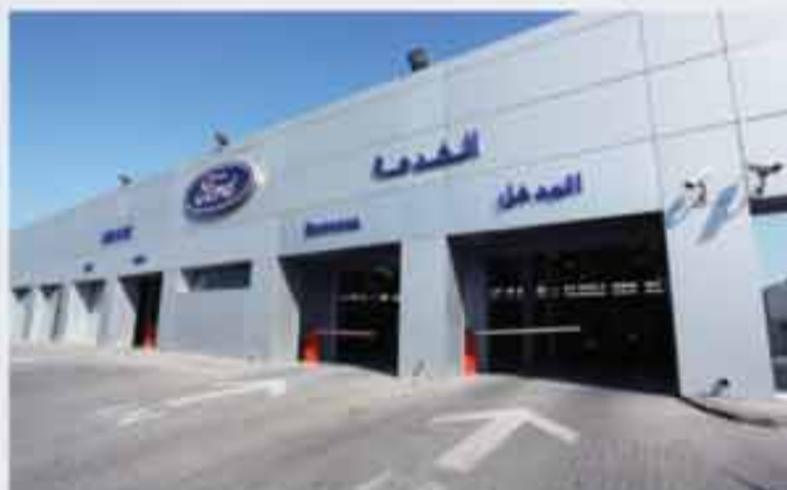
Vehicle entrance at the new Service Center
