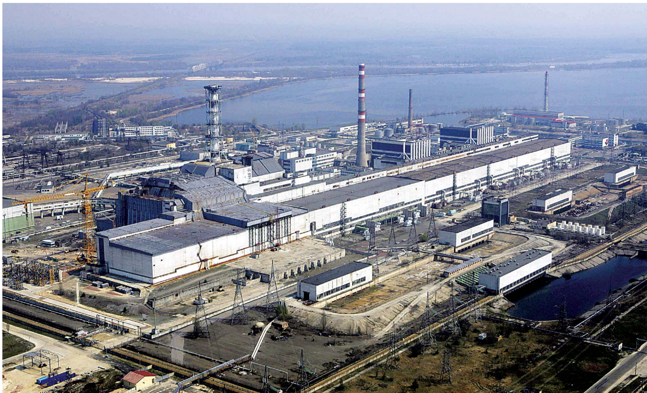
An aerial view shows the Chernobyl nuclear power plant in Ukraine on April 26, 2006. From the air, one can see the damaged reactor encased in cement and steel, image left, put in place after the 1986 explosion to cut down on radiation leaking into the environment. —AP
