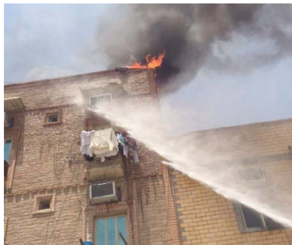
Flames coming out from a traditional Arab-style house in Khaitan.
