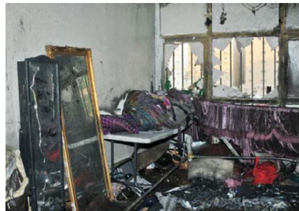
Severe damage left by a fire inside a Jahra apartment.
