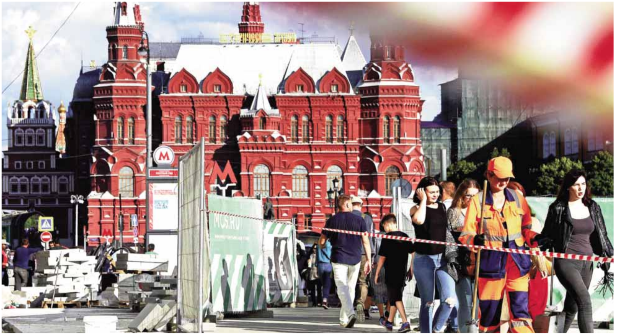
MOSCOW: People walk past construction works in central Moscow on July 11, 2016. — AFP
