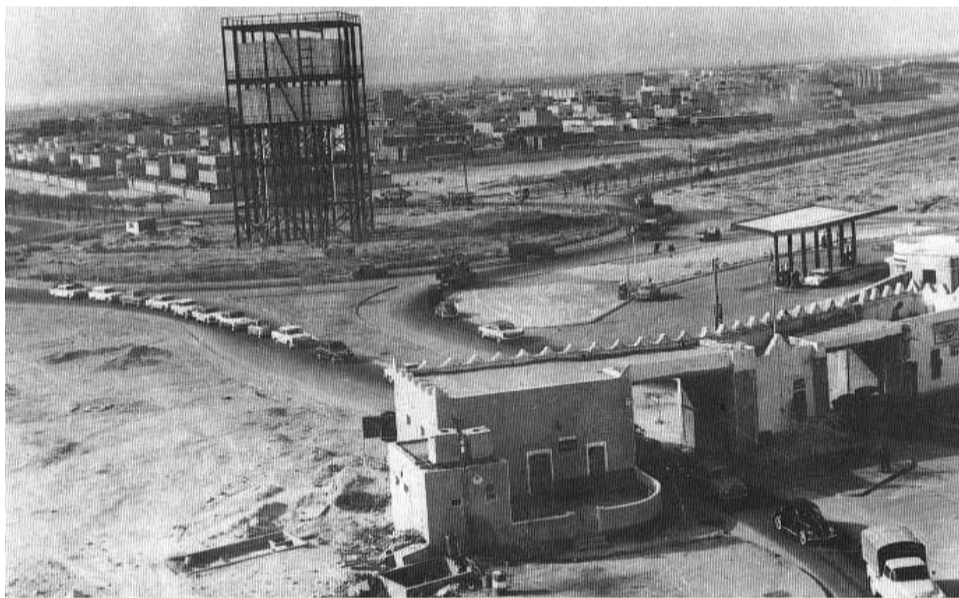
An aerial view of the wall
