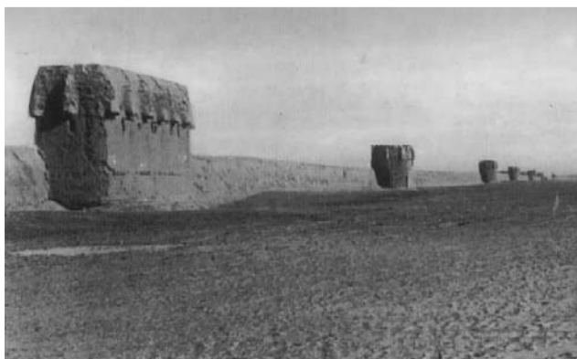
The third wall of Kuwait, built in the 1920s which is an embodiment of solidarity between the leadership and people of the land.
