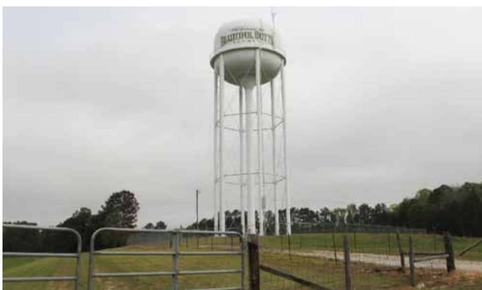
A water tower is seen in Butts County, GA. Named for Capt Samuel Butts, who died in 1814 during the Creek War, residents at one point suggested a name change.
