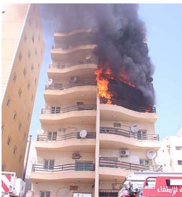
Flames come out of an apartment in Salmiya yesterday.
