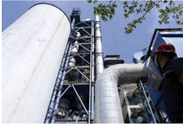
HANDAN: A worker looking at a cement plant in Handan, in China's northern Hebei province. China's economy expanded at its slowest rate in seven years during the first quarter, the government said on April 15, but forecast-beating readings for March raised hopes a growth slowdown in the Asian giant may be bottoming out. — AFP
