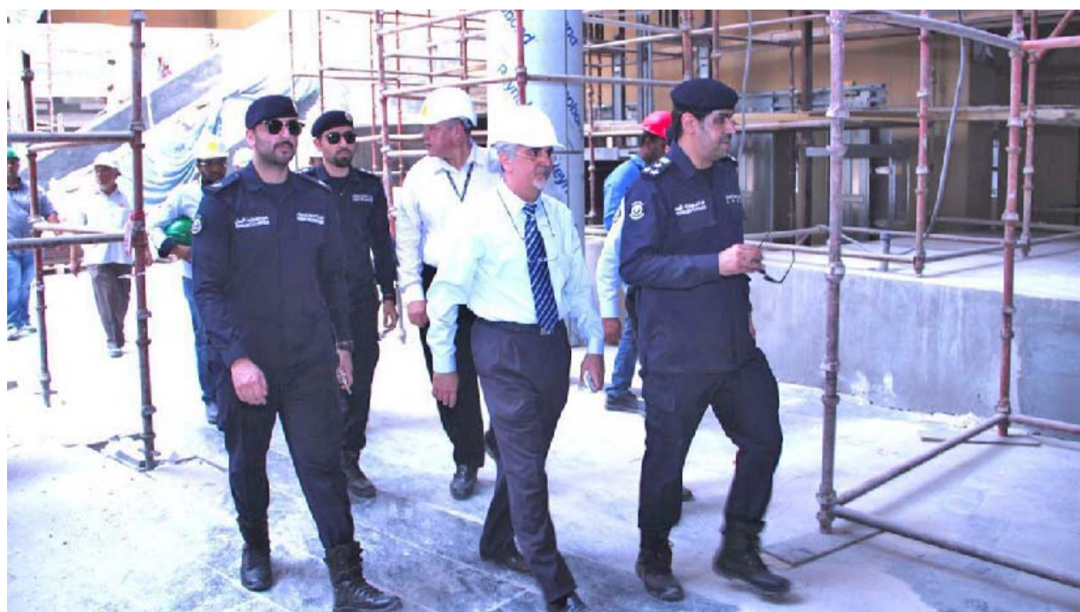
KUWAIT: A team from the prevention sector inspected safety and fire prevention equipment in the education ministry diwan building project in South Surra. — By Hanan Al-Saadoun
