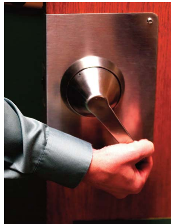
OSAWATOMIE: Osawatomie State Hospital superintendent John Worley demonstrates ligature proof door handles during a tour of the state hospital grounds in Osawatomie, Kan. Officials and consultants are improving staffing and overhaul hospital operations so that it can regain federal certification. — AP
