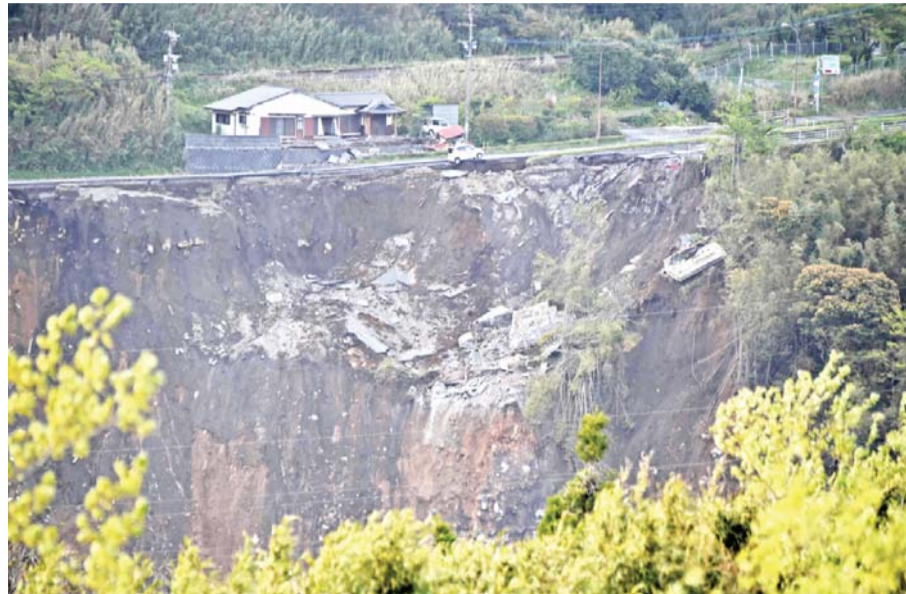
TOKYO: This picture shows a collapsed road in Minami-Aso, Kumamoto prefecture yesterday. At least 41 people are known to have died in the double disaster, with up to eight still missing - feared buried in shattered houses or under torrents of mud. — AFP
