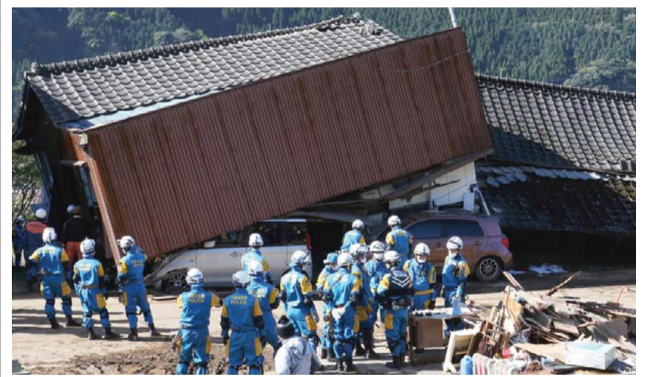
MIMAMI-ASO, Japan: Rescue workers try to save people from a collapsed house in this town in Kumamoto prefecture yesterday. — AFP
