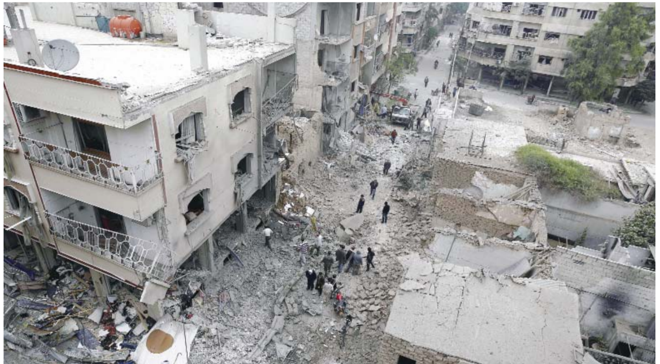
DOUMA, Syria: Syrians inspect damaged buildings following an air strike by Syrian government forces in this rebel-held area east of the capital Damascus. — AFP
