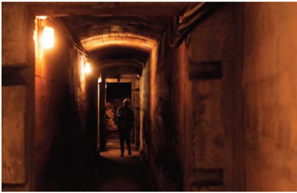
Photo shows a reinforced tunnel and an unfinished lift shaft under Książ Castle.
