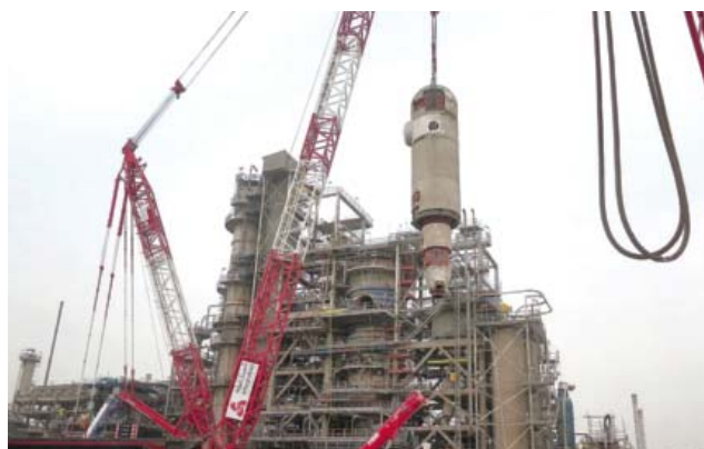
The new Fluid Catalytic Cracking Unit installation process.
