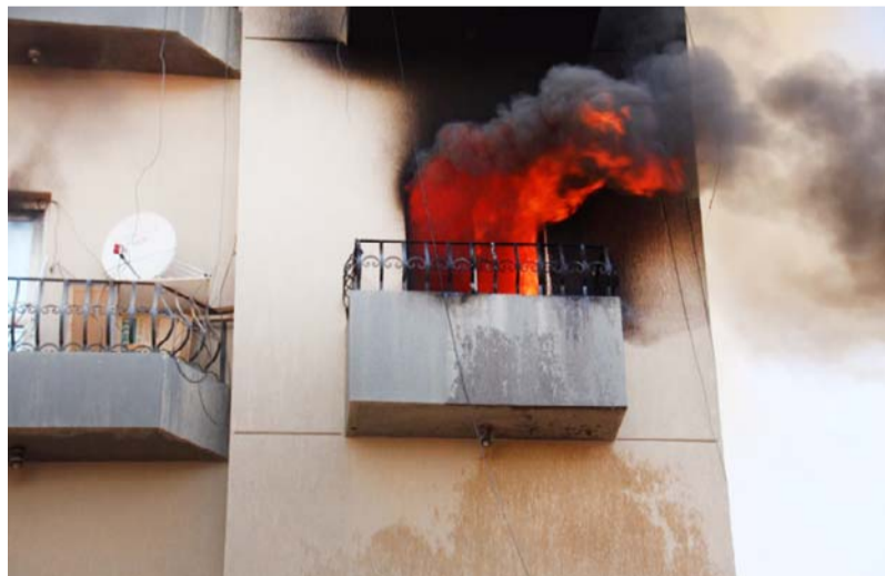
Flames coming out of an apartment's window in Hawally.
