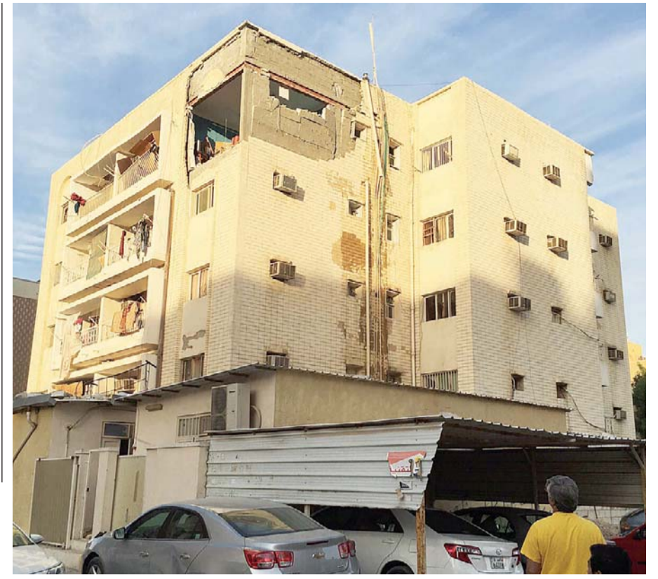
KUWAIT: The picture shows a fourth-storey apartment heavily damaged following an explosion yesterday.
