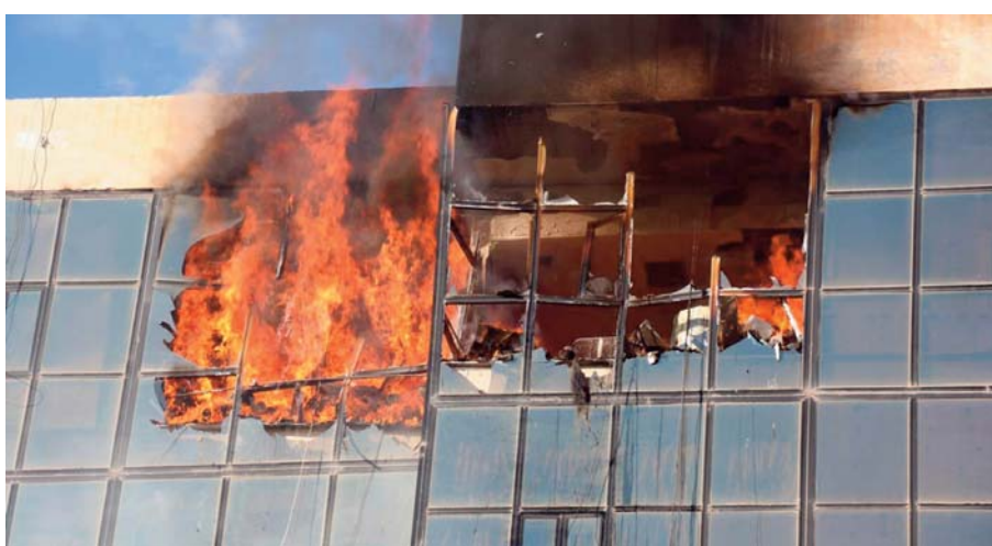
KUWAIT: A fire broke at an apartment located in the Arbeed apartment buildings in Rega'ie yesterday. Firefighters managed to put the blaze under control before it could spread to other apartments. Three firemen were injured and were treated at the scene. Meanwhile, a case was filed to investigate the cause of the fire. — By Hanan Al-Saadoun
