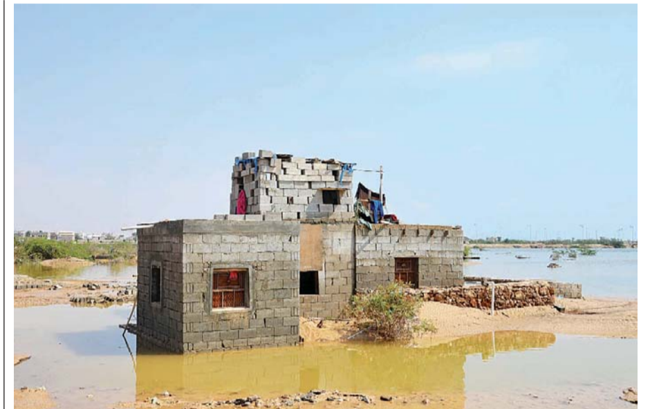
MUKALLA: Water surrounds a Yemeni home following a tropical cyclone that has slammed into the war-ravaged country, in Mukalla in Yemen's Hadramawt province. Packing winds of more than 100 kilometers per hour, Cyclone Chapala made landfall in the southeastern provinces of Hadramawt and Shabwa, Minister of Fisheries Fahd Kafain said. —AFP
