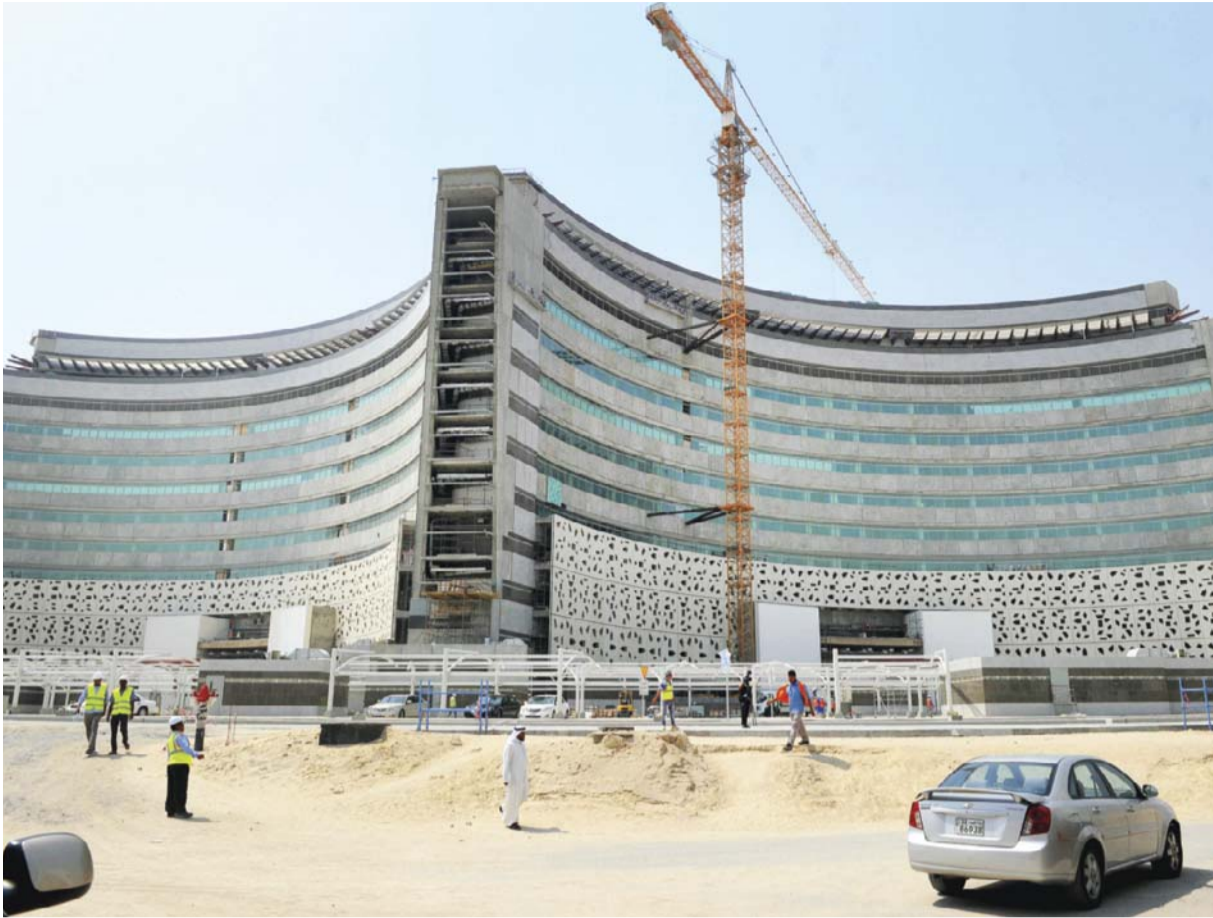
Final stages of construction at the Jaber Hospital.
