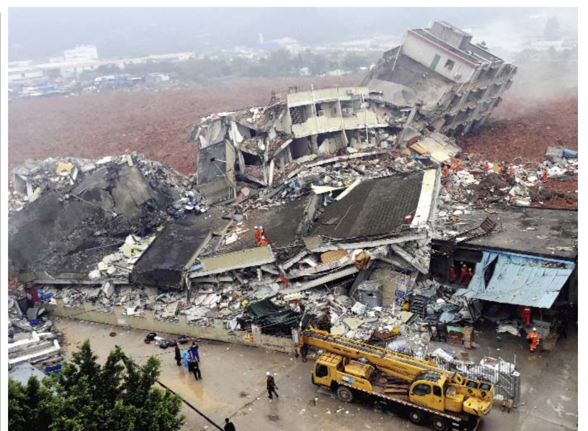
SHENZHEN: Rescuers search for survivors amongst collapsed buildings after a landslide in south China's Guangdong province yesterday. The landslide collapsed and buried buildings at and around an industrial park in the southern Chinese city of Shenzhen on Sunday authorities reported. — AP
