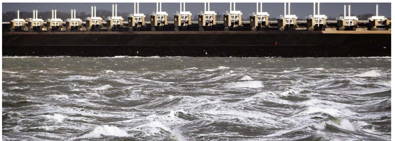
High water at the Eastern Scheldt storm surge barrier (Oosterscheldekering) in Oosterschelde. Had nature been left to take its course much of the Netherlands would be a muddy swamp and the tiny coastal nation would never have risen to be the euro-zone's fifth largest economy. — AFP
