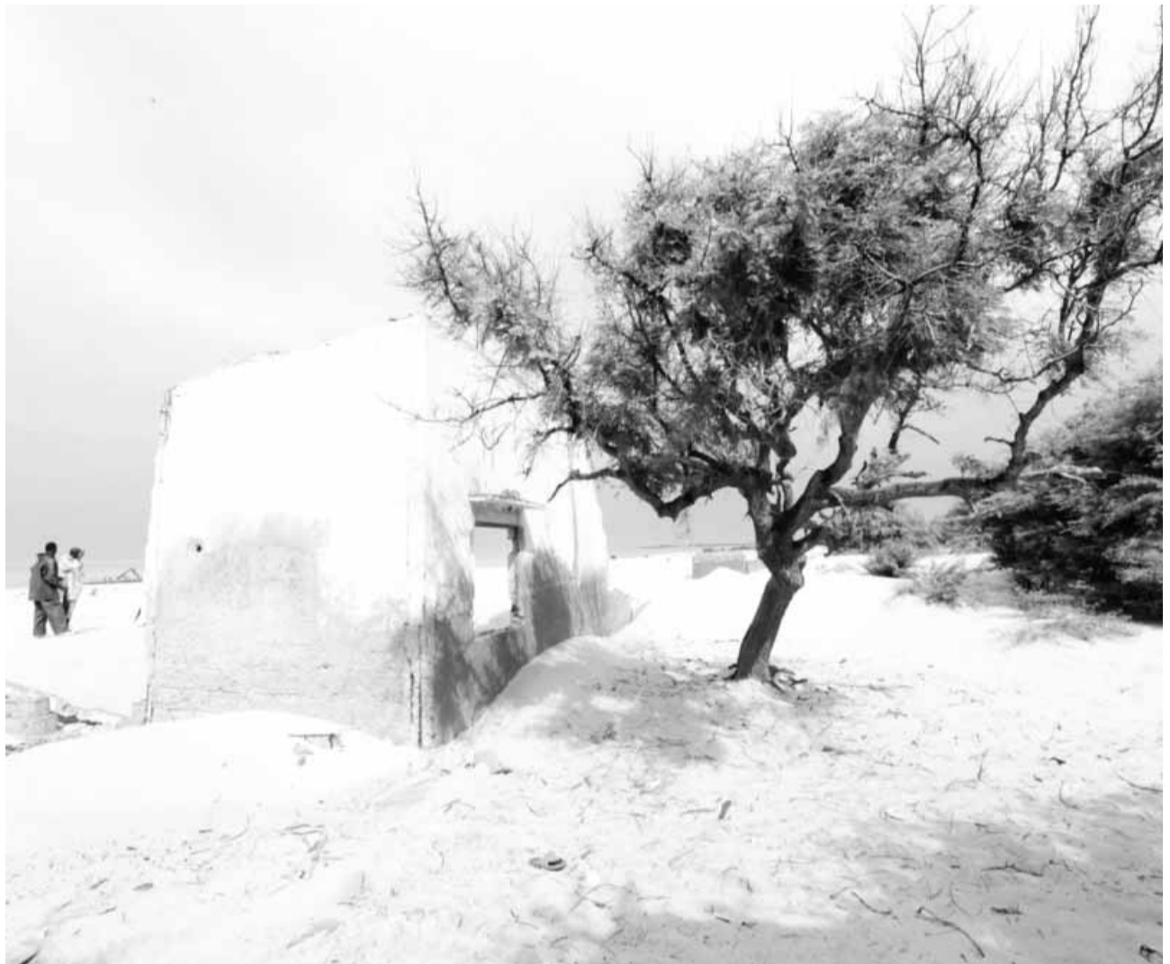
SAINT-LOUIS DU SENEGAL: Near Saint-Louis du Senegal shows the remains of a house of the Doune Baba Dieye village which was abandoned because of the approaching sea. — AFP
