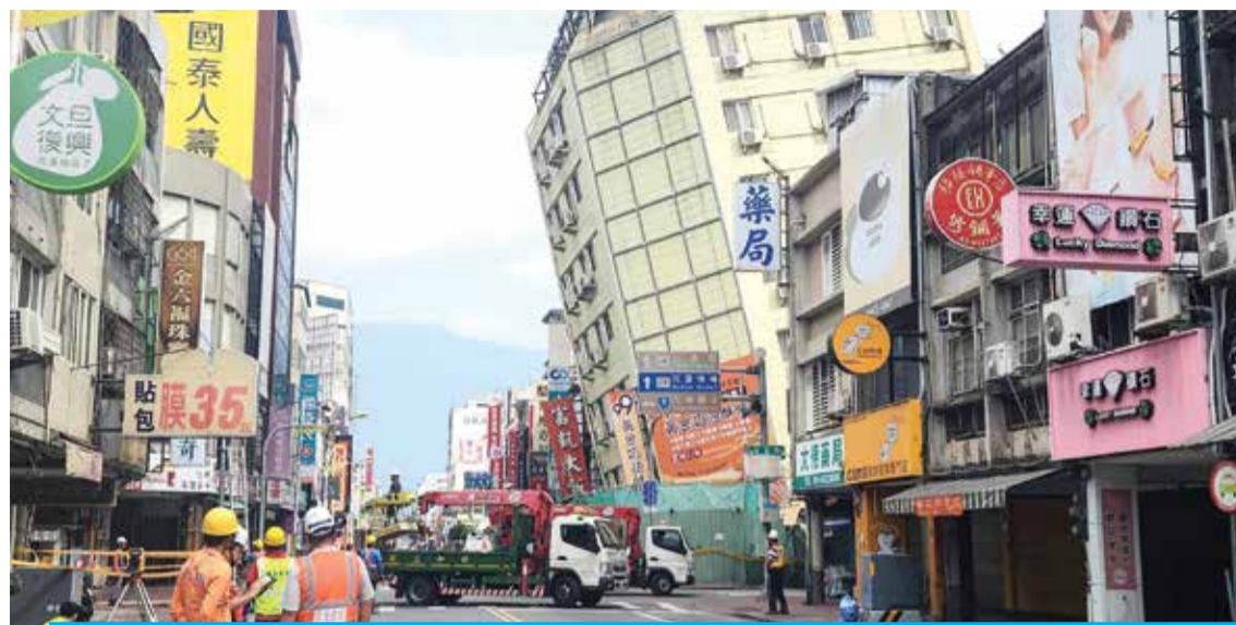
HUALIEN, Taiwan: This picture shows the Full Hotel building, which had been previously damaged in the April 3 earthquake, tilting further to one side on April 23, 2024, after a series of earthquakes overnight. - AFP
