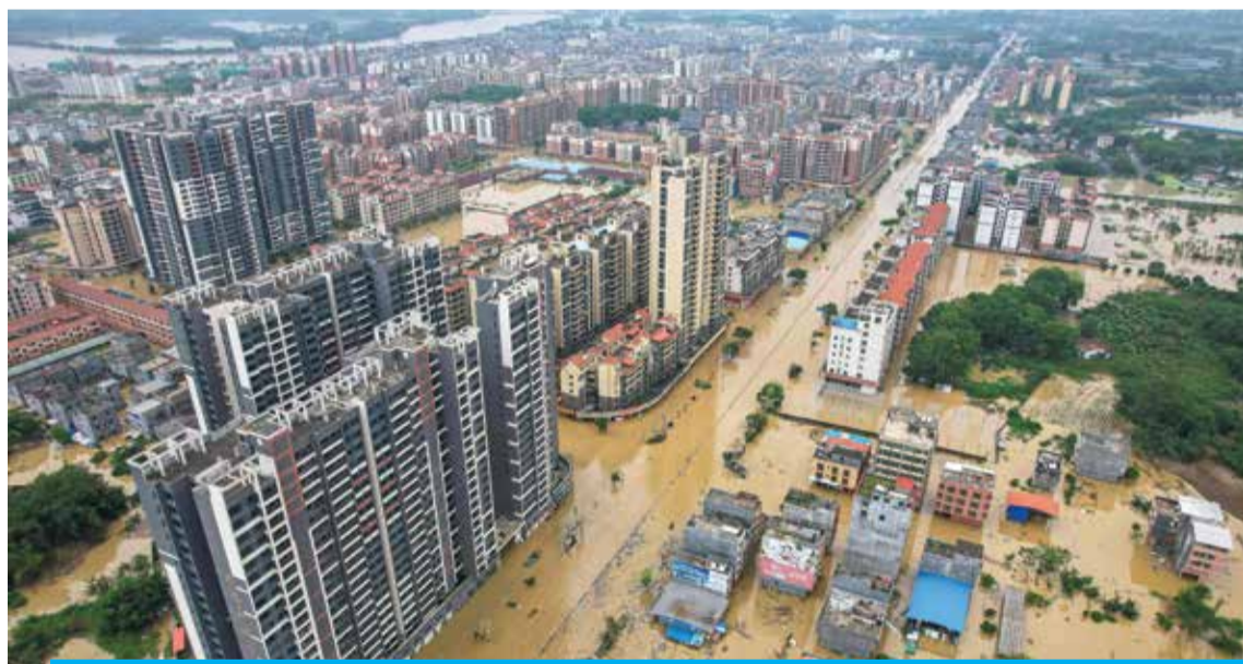
QINGYUAN, China: This aerial photo taken on April 22, 2024 shows a general view of flooded buildings and streets after heavy rains in this city in the southern Guangdong province. — AFP
